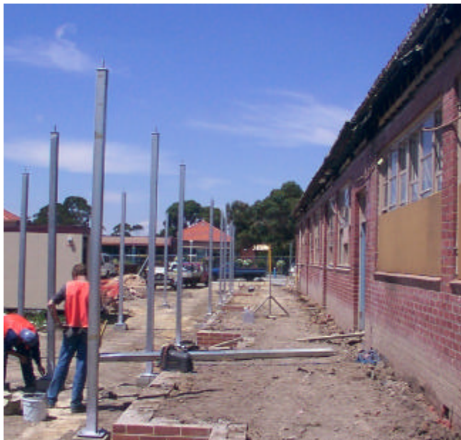
PREPARATION FOR THE NEW VERANDAH ON THE NORTHERN SIDE
